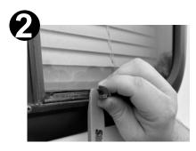
Remove the old window edge trim by gently pulling it out of the window frame track. If an adhesive or calking has been used, take care to remove this as well and clean the track thoroghly.
